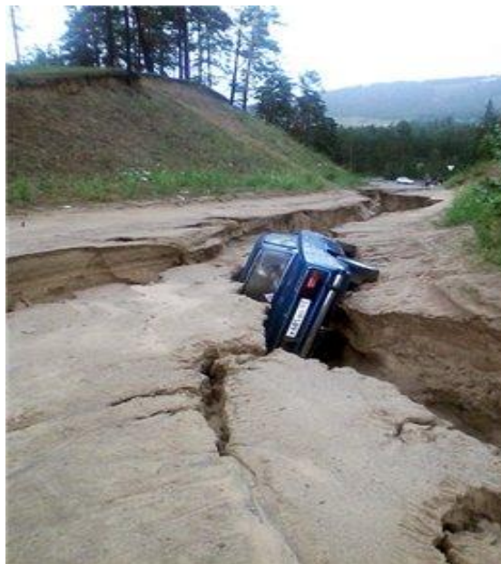
Pic. 11. Washout of road.
