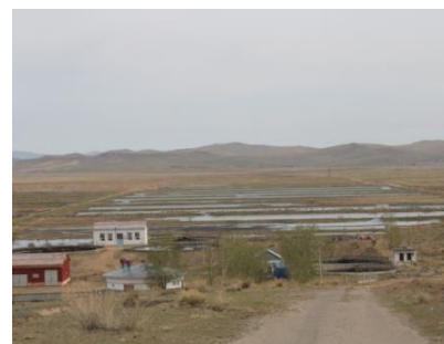
Figure 22. The Darkhan Wastewater Treatment Plant
