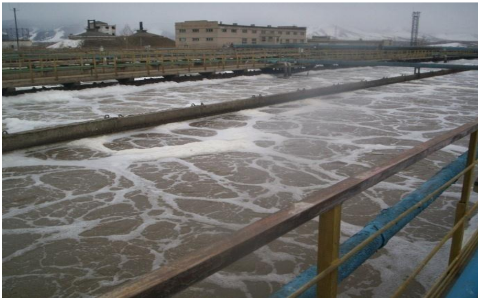
Figure 4.4.2.c The central wastewater treatment facilities of Ulaanbaatar, Mongolia. Photo: G.Tamir.
