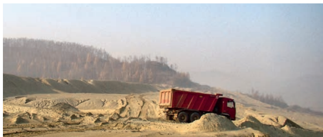
Pic. 4.3.9 Relocation of sand from the Modonkul river valley into a former hydraulic dump.
