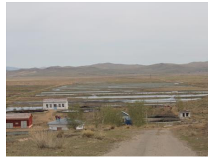
Figure 22. The Darkhan Wastewater Treatment Plant
